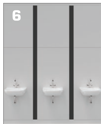
6. Install the remaining cladding.
